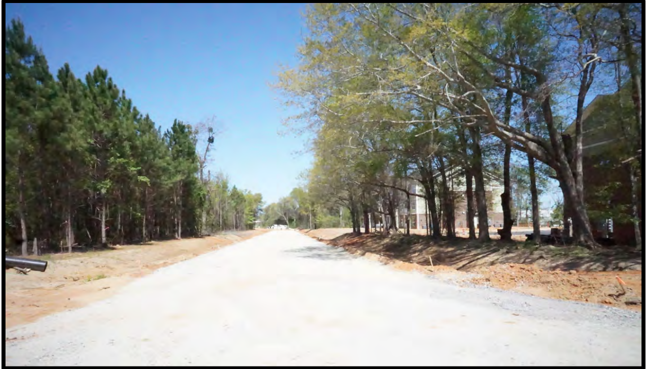
Photo 3 – road being built at the western side of the site
